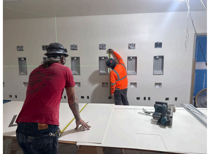
Bouten Construction installing FRP within the laundry room.
