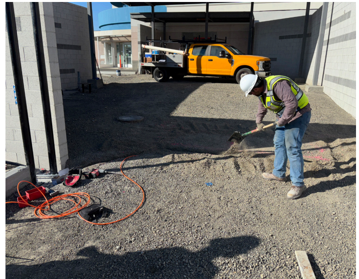
Northwest Fencing installing the electrical loop for sallyport gates.
