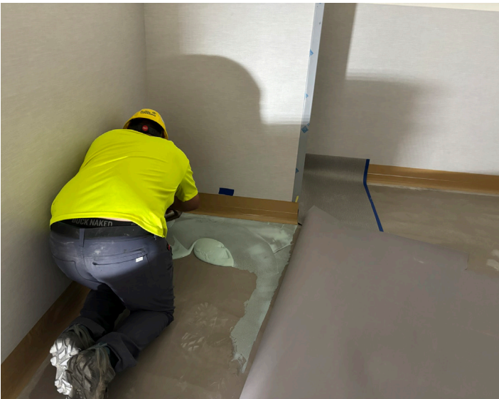
Standard Paint & Floor installing sheet vinyl within Assessment & Exam.
